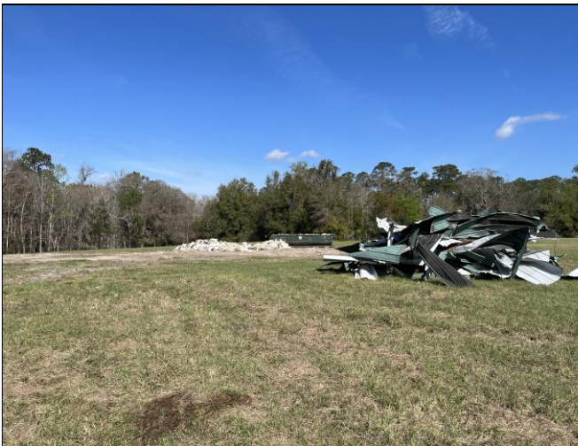
Demolished pole barn near northwesterly end of parcel
